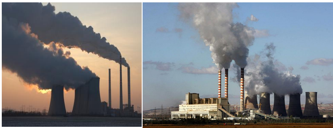
Figure 7. The Ptolemaida power stations. The area Florina-Amintaiio-Ptolemaida-Kozani with 1.82 billion tons of lignite has the 57% of exploitable reserves and 79% (2006) of lignite production came from Western Macedonia.
